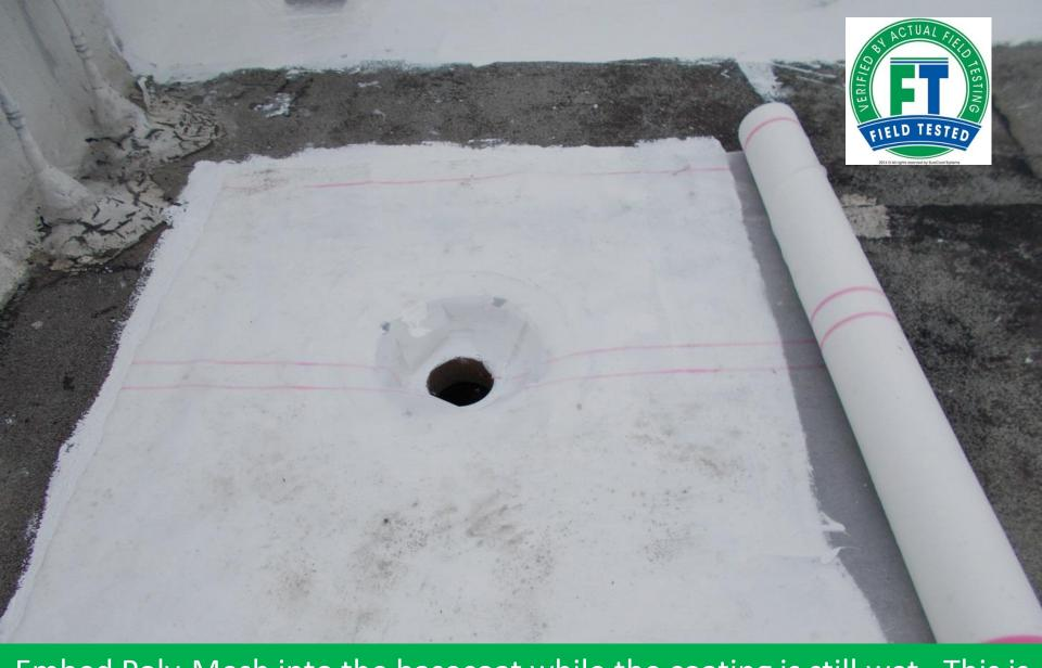
Embed Poly-Mesh into the basecoat while the coating is still wet. This is for added tensile strength. A SureCoat roof drain repair will have a 2800 psi tensile strength when reinforced with Poly-Mesh.
