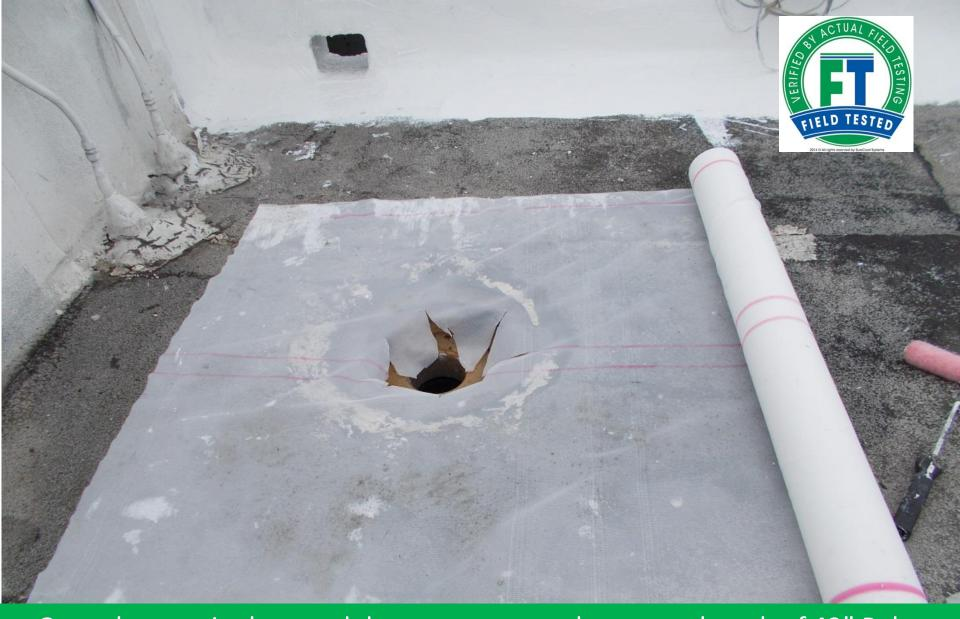
Once the area is clean and dry, measure out the proper length of 42" Poly-Mesh, extending 2-3 feet on each side of the roof drain. Cut out a hole in the center allowing the Poly-Mesh to fold into the roof drain.
