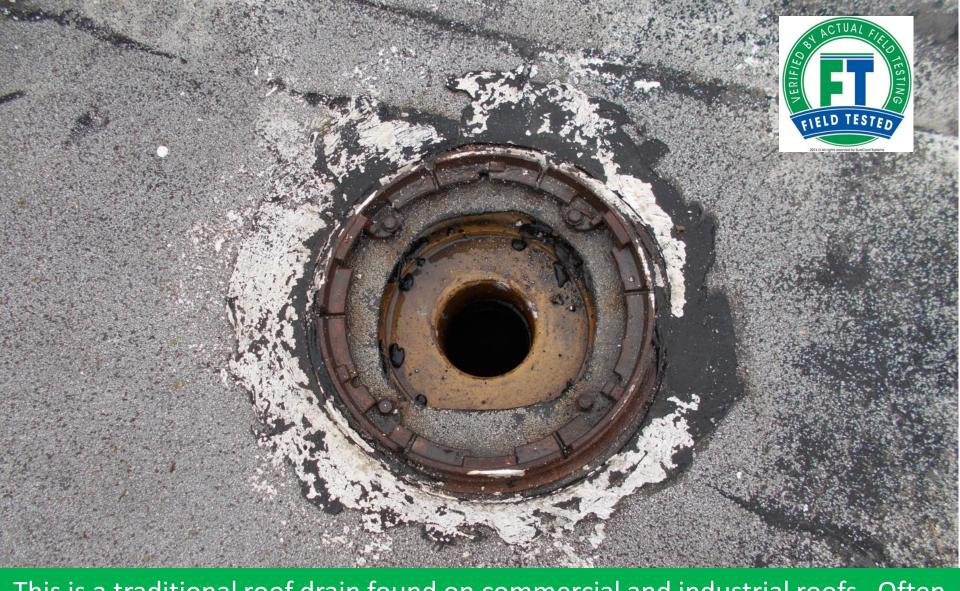
This is a traditional roof drain found on commercial and industrial roofs. Often roof leaks occur at the roof drains. This roof drain has been repaired several times with mastic and inferior coating products that were unable to withstand the UV exposure and ponding water common near roof drains.
