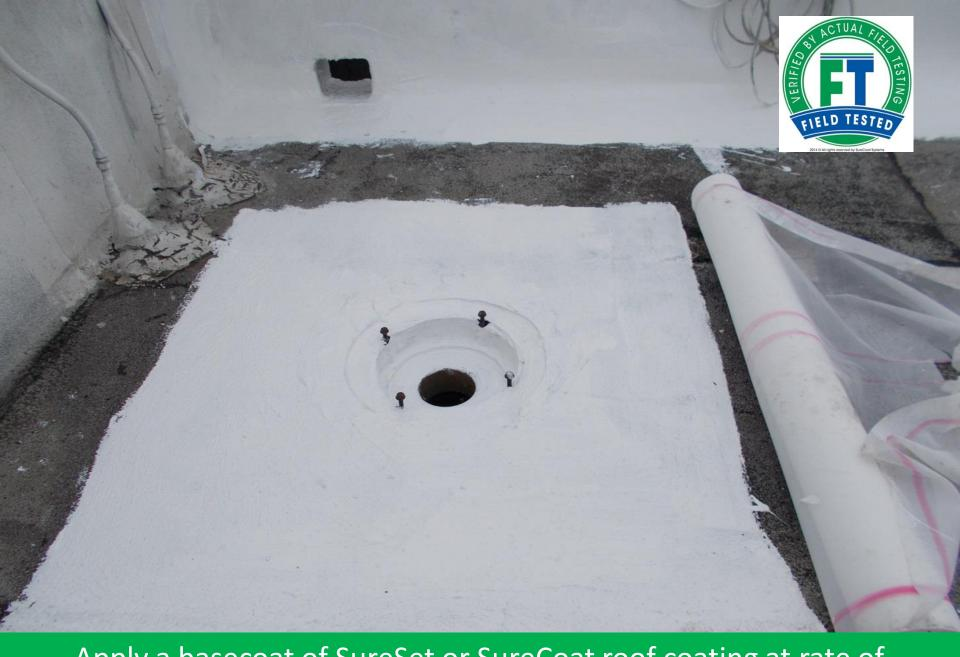
Apply a basecoat of SureSet or SureCoat roof coating at rate of approximately 20 mils or 2 gallons per SQ (100 SF).
