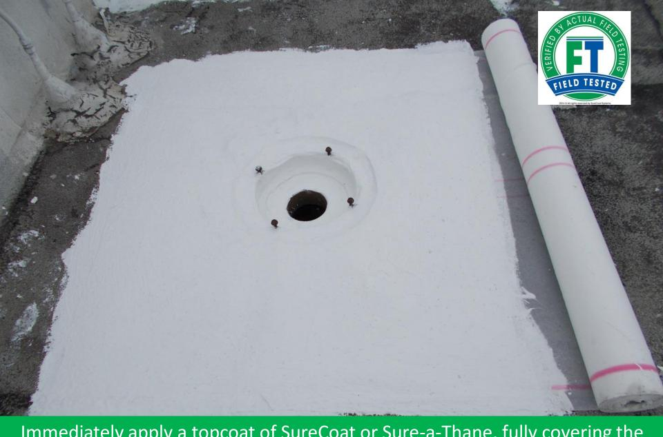
Immediately apply a topcoat of SureCoat or Sure-a-Thane, fully covering the Poly-Mesh, forcing the basecoat to bleed through and fully covering the Poly-Mesh. Extend the topcoat of coating beyond the Poly-Mesh a minimum of 12".
