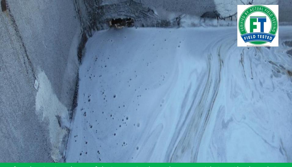
Before beginning the roof drain repair, clean the area with SureSkrub and rinse thoroughly. Flat and low-sloped roofs often have ponding water around the roof drains as shown above. Ponding water causes accelerated deterioration of traditional roofing materials. The SureCoat Roof System protects against ponding water!
