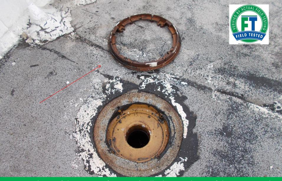
Remove the roof drain ring. If not too badly damaged, a roof drain ring can be cleaned using SureSkrub to remove the surface rust then treated with a rust inhibitor and painted or coated. Maintaining the roof drain ring is important
