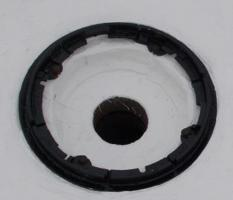
There should not be any Poly-Mesh visible through the coating once complete. Make sure the entire areas is pin-hole free and dry throughout. Then, secure the roof drain ring back in place.
