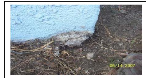
3. **Clean** surfaces by using a power washer to remove all dirt, loose stucco, paint and mold. Be careful not to use too much force and unnecessarily remove stucco or paint.
