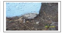
3. Clean surfaces by using a power washer to remove all dirt, loose stucco, paint and mold. Be careful not to use too much force and unnecessarily remove stucco or paint.
