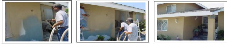
8. Apply *StrucSureCoat* to the fascia boards and other wood trim areas with a paintbrush. You can also use an airless to spray the soffit and trim areas. **\*\*Touch ups should be done from corner to corner on any surface for uniform appearance.**
